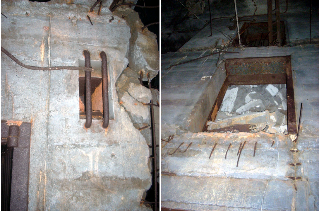
Figure 10. C.I.C. building: a) damages in the third underground floor; b) damages to the second and first underground floors seen from the third underground floor
