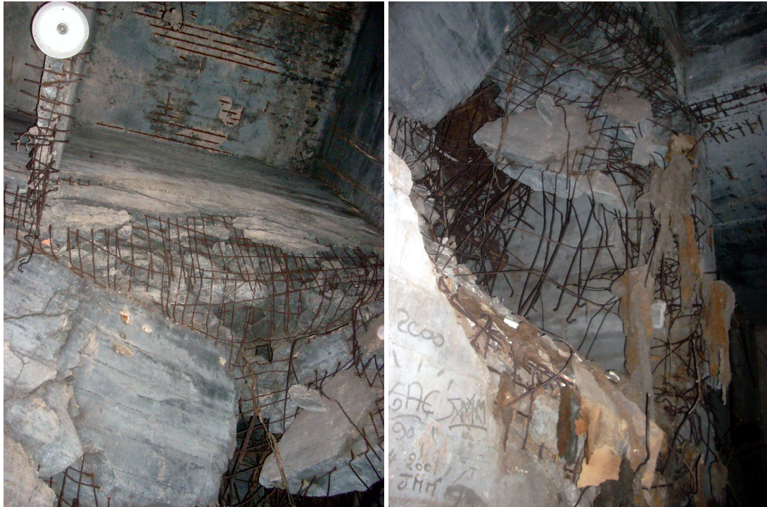
Figure 8. C.I.C. building: a), b) damages in the second underground floor seen from the third underground floor
