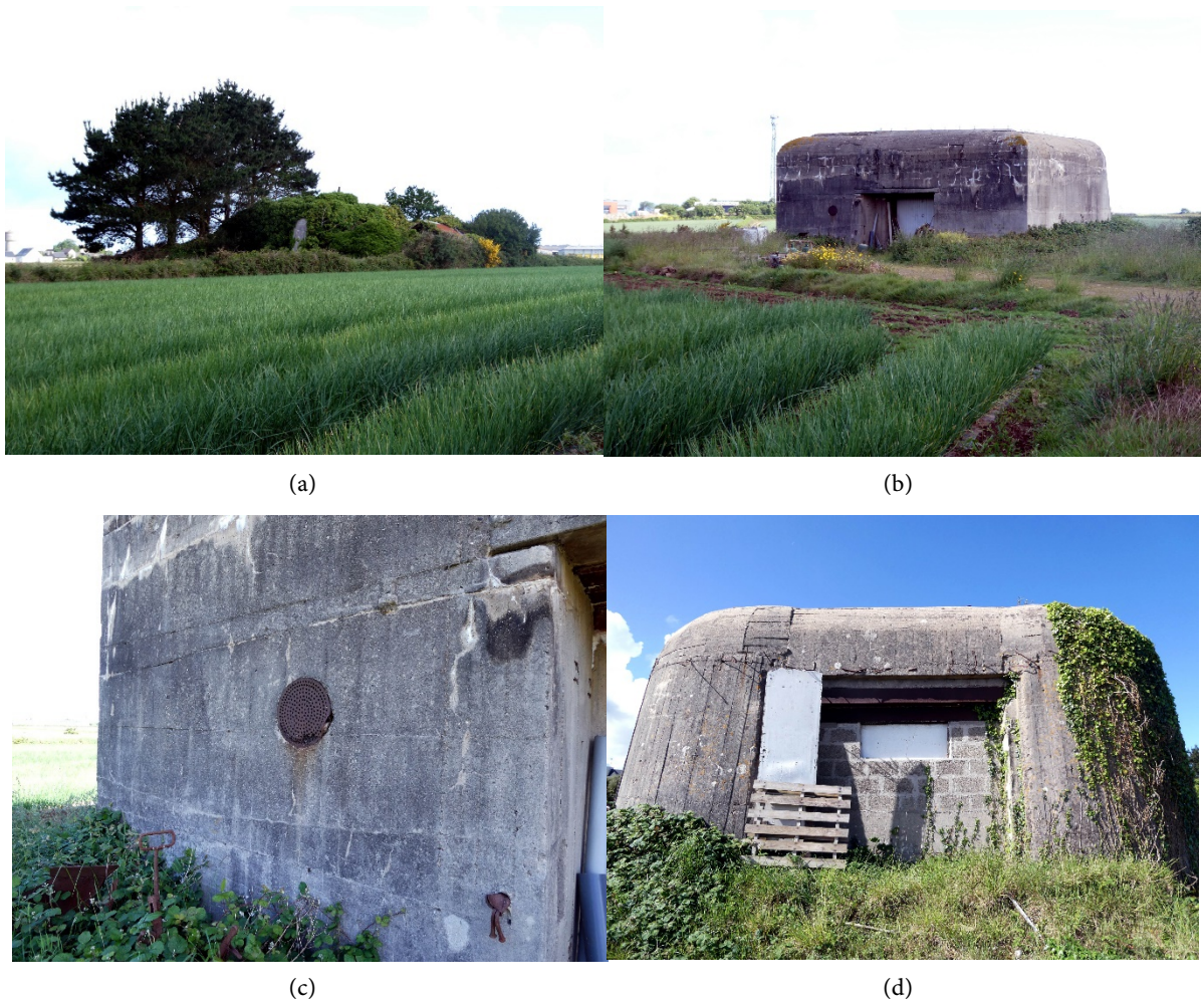
Figure 6. (a) R 669 (3); (b) R 669 (4) rear side; (c) R 669 (4) grid of the exhausted combat gas pipe; (d) R 669 (4) front side.
