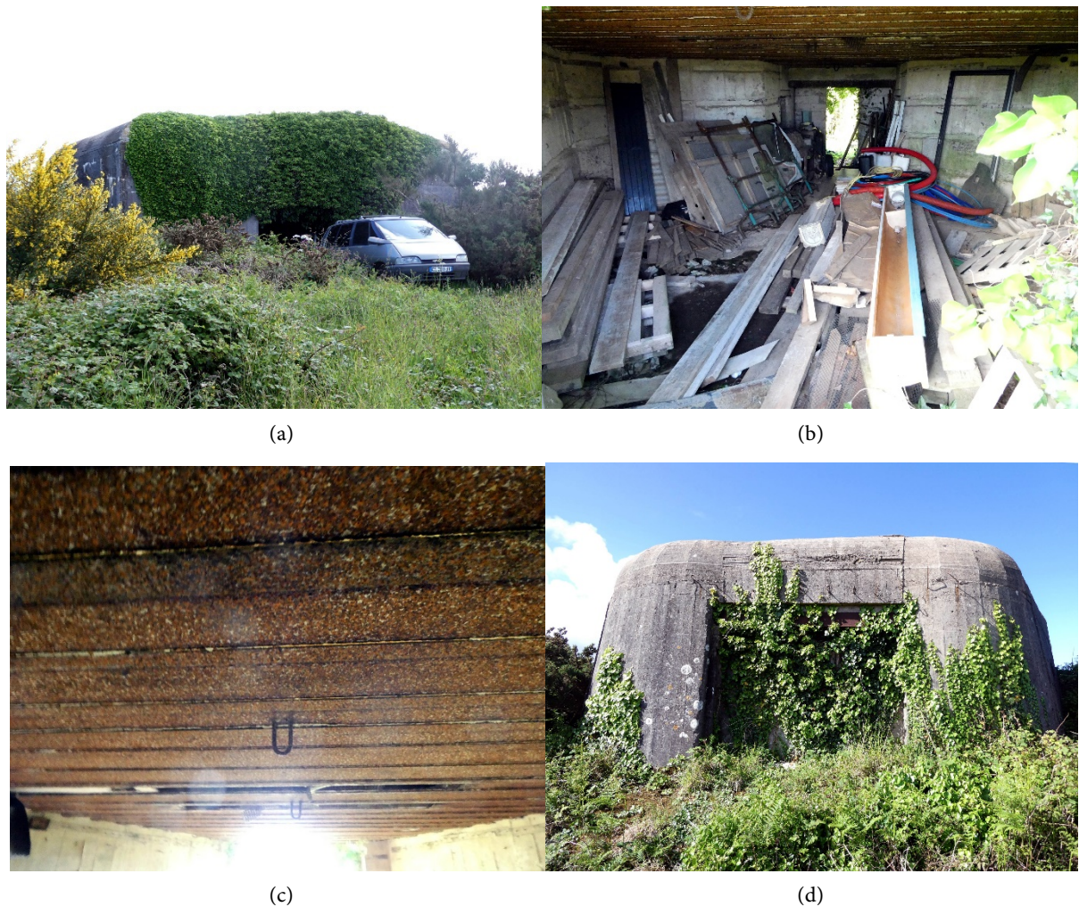
Figure 7. (a) R 669 (5) rear side; (b) R 669 (5) interior, (c) R 669 (5) rusted ceilings with two gun lifting joints and two elongate gates of the combat gas extraction system; (d) R 669 (5) front side.
