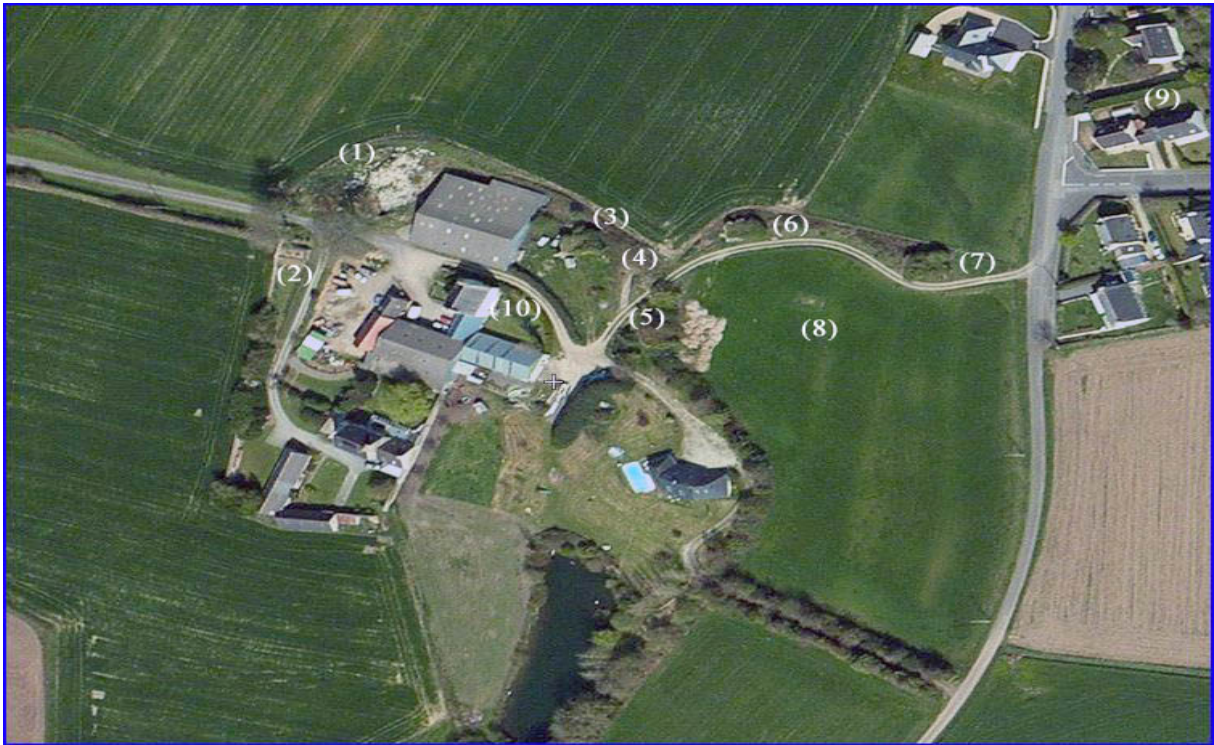
Figure 12. Stp Av 55 : general plan: (1) dismantled H 671 , (2) one room bunker, (3) H 671 , (4) one room bunker, (5) one room bunker, (6) H 671 , (7) H 671 , (8) place of two bunkers buried in the terrain, (9) Plouider, (10) farm (Tomezzoli, 2016) [Flash Earth].
