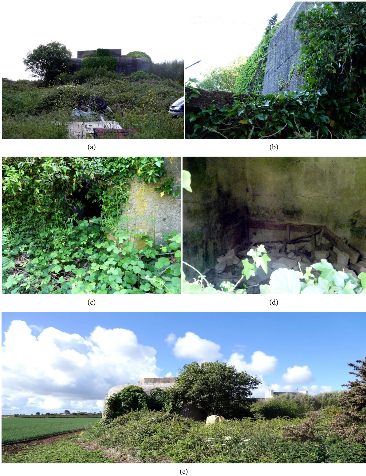
Figure 8. (a) R 669 (6) with Flak emplacement, rear side; (b) R 669 (6) and annexed construction, (c) Annexed construction entrance; (d) annexed construction interior; (e) R 669 (6) front side.
