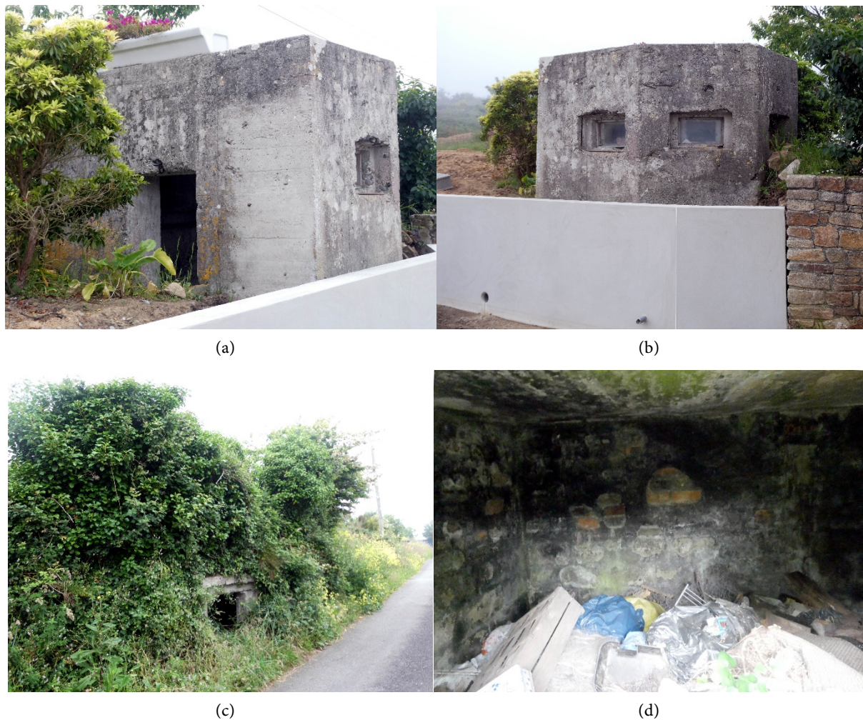
Figure 4. (a) Pentagonal watch post rear side; (b) Pentagonal watch post front side; (c) One room bunker (14) entrance; (d) One room bunker (14) internal room.
