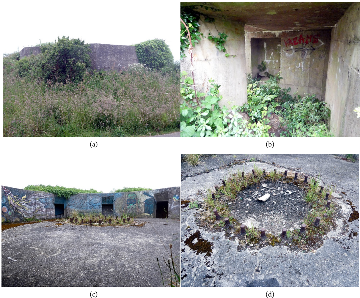
Figure 3. FI 243b : (a) External view; (b) Labyrinth entrance with rectangular niche; (c) Open gun emplacement; (d) 21 screws ring.
