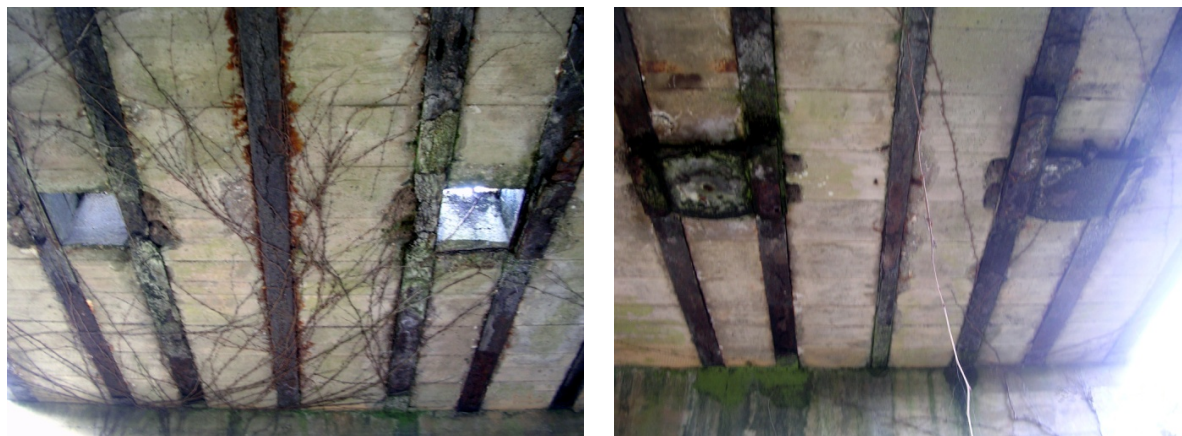
Figure 4. Kieswerk: first silo—opened and closed hoppers on the loading way.
