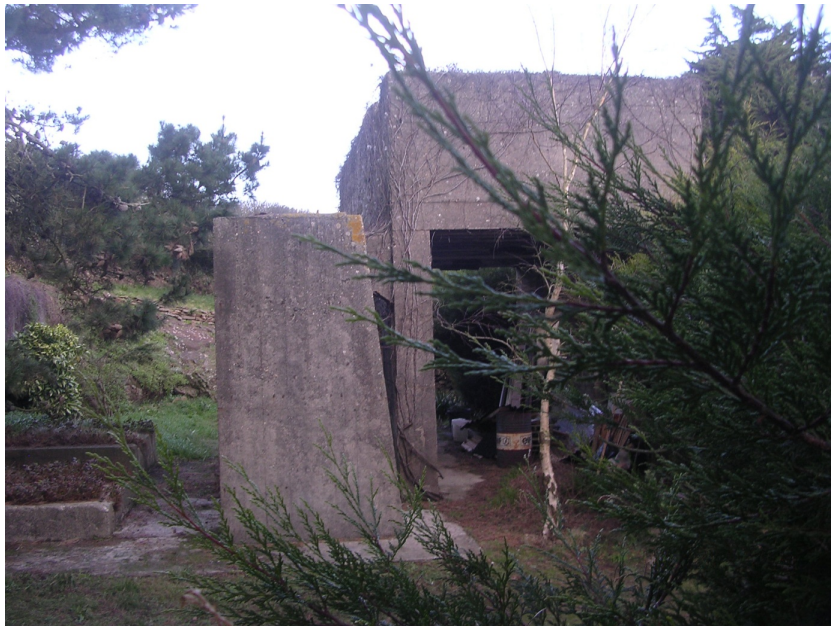
Figure 5. Kieswerk: first silo—concrete support of the loading conveyor belt mechanism.
