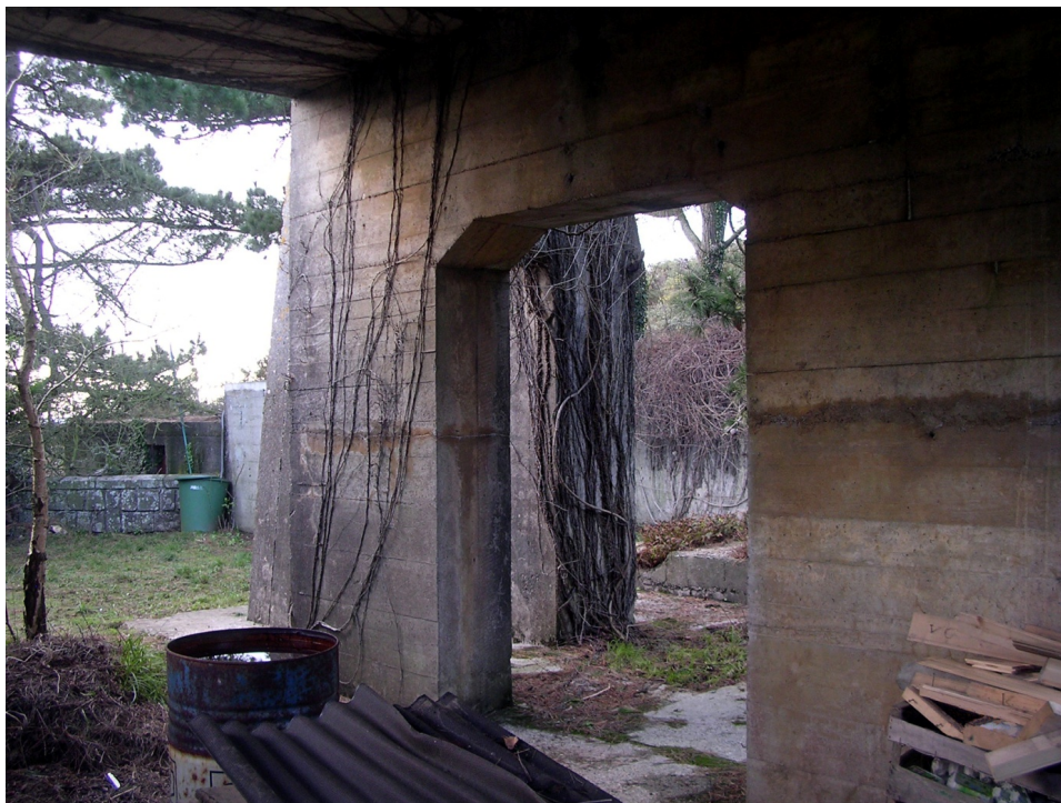
Figure 3. Kieswerk: first silo—loading way.
