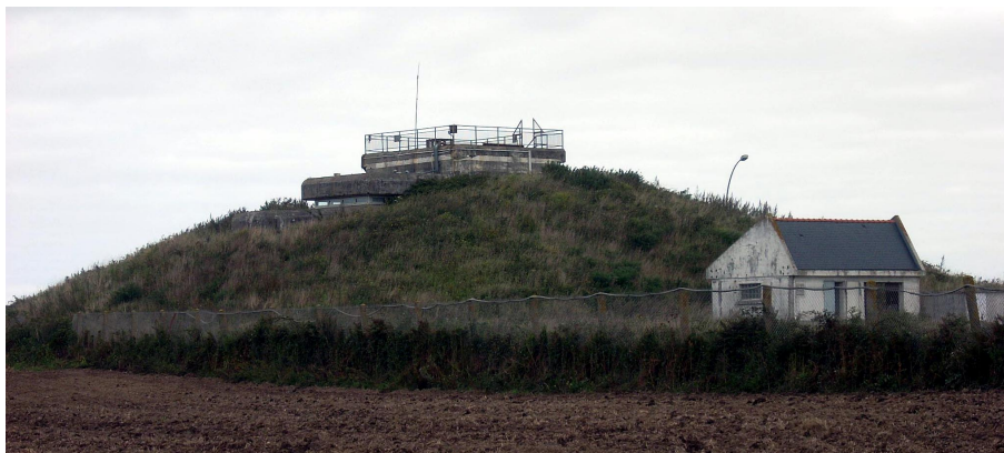
Figure 7. RE 302 MKB Graf Spee—fire control bunker S 414.
