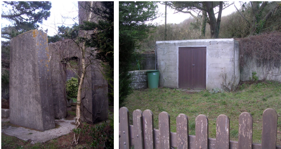
Figure 6. Kieswerk: first silo concrete supports of the loading conveyor belt mechanism and concrete barrack.
