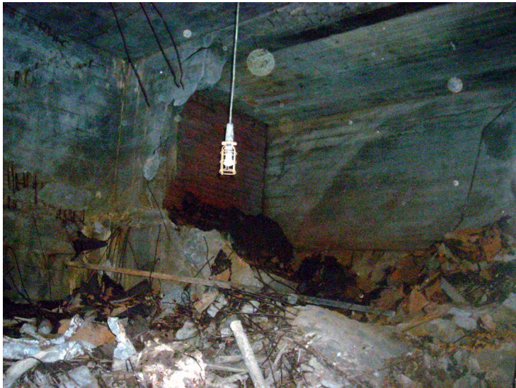
Figure 11. C.I.C. building: damages in the third underground floor.
