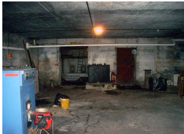
Figure 4. C.I.C. building: first underground floor—rooms of the heating system and fuel tanks disappeared, on the left side the modern gas heating system.
